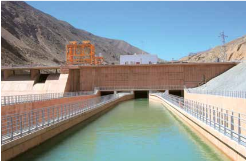
Cheves Hydropower Plant, operated by Statkraft Peru
